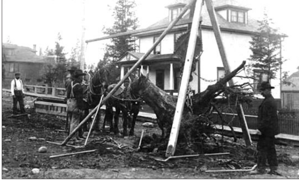
Stump pullers at work, ca. 1907, on the 200 block of 11th Avenue. Prisoners from the local jail were often engaged for such tasks.
